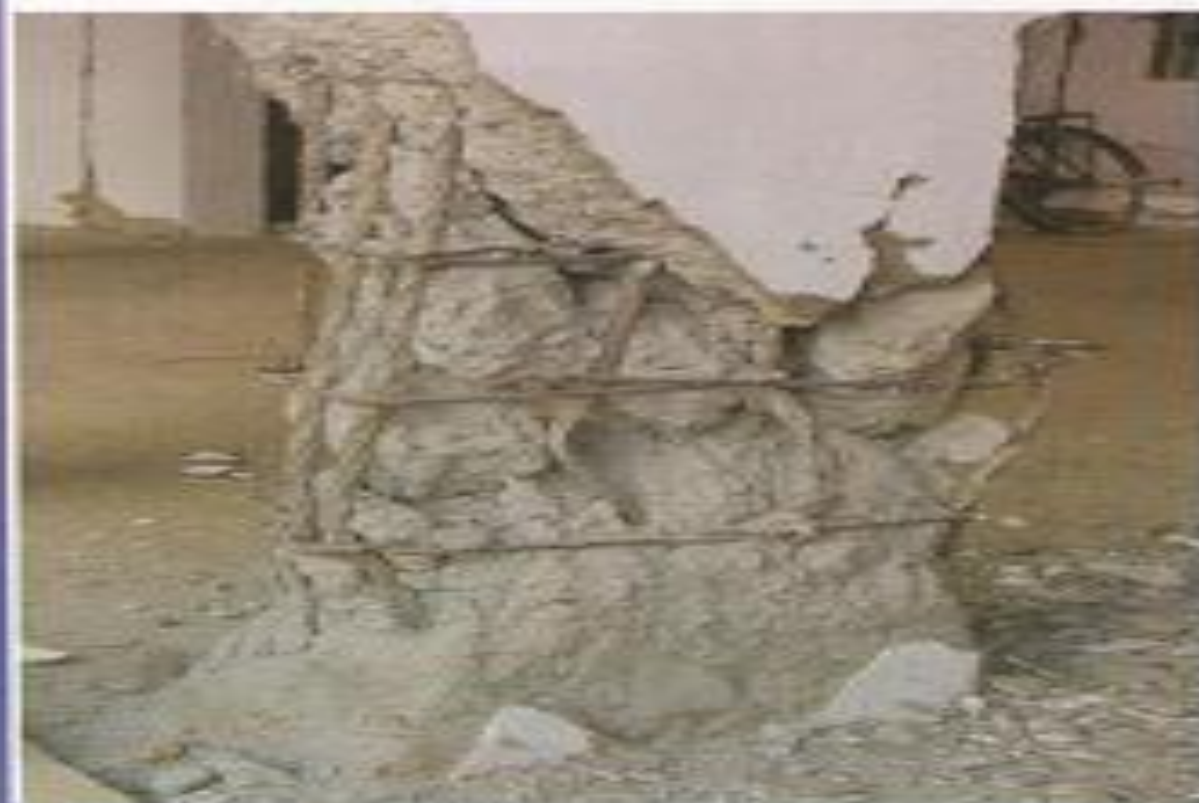
Figure 2: Steel reinforcement in seismic columns – closed ties with 135^\circ hooks are required as per Indian Ductile Detailing Code IS:13920-1993.
